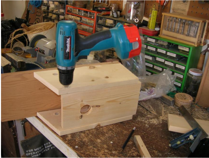
Drill pilot hole for 1 1/2 inch #8 deck screw to hinge front
